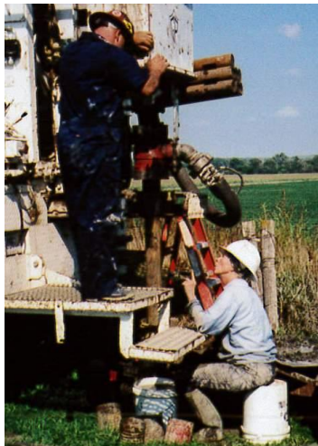
Matt Marxen and Sue Lackey, UNL-CSD drilling a test hole in the Lewis & Clark NRD.
